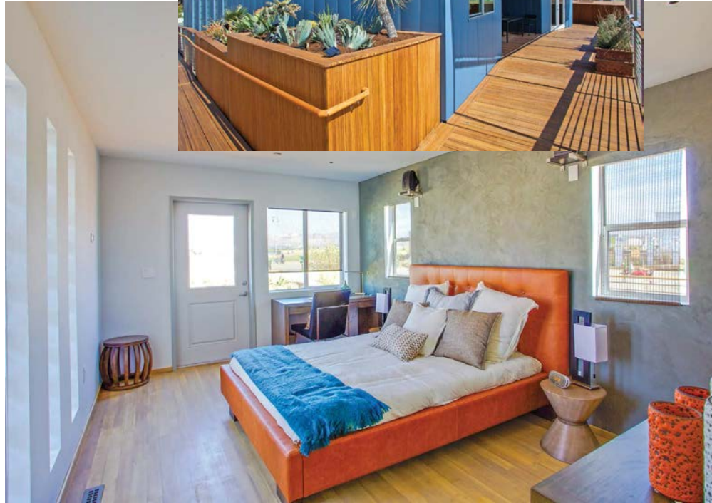
A coating of earthen clay on the interior of the wall behind the bed helps keep the bedroom cool by absorbing and releasing moisture based on indoor humidity levels.
