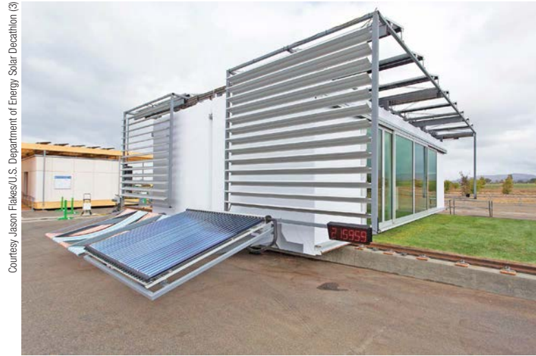
Southern California Institute of Architecture and California Institute of Technology's solar hot water system consists of evacuated tubes on an innovative mounting system.
