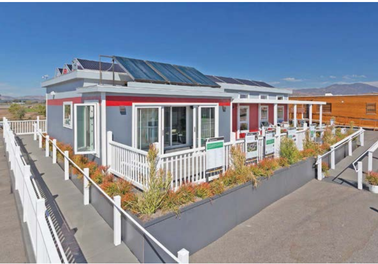
Flat-plate solar collectors on the Missouri University of Science and Technology's house helped it tie with six other teams for first place in the hot water contest.
