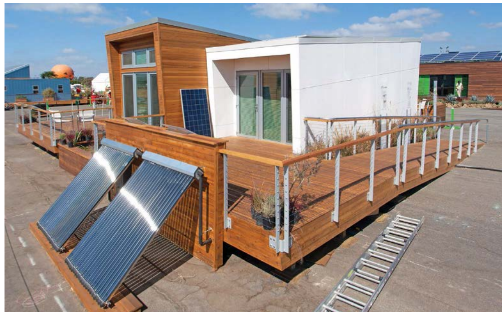
The University of Calgary's Team Alberta home was another that used evacuated-tube collectors to meet its water-heating needs.
