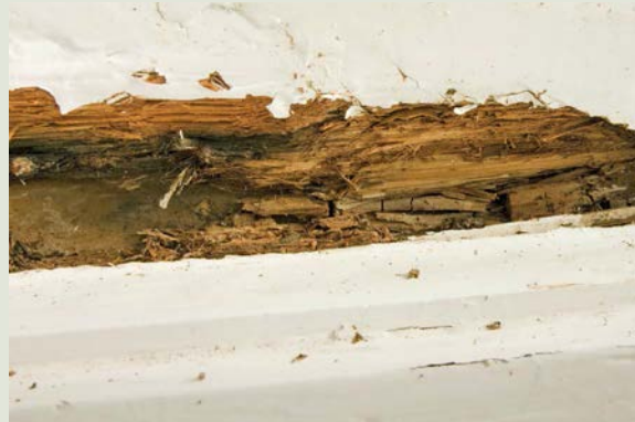
When wooden window frames have degraded to this degree, it's time to consider replacement.
