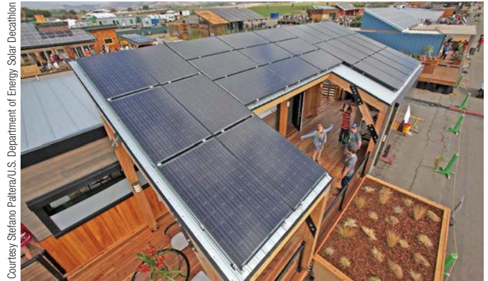
The sloped exostructure of Team Ontario's house accommodates a flush-mounted PV array.
