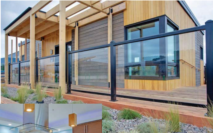
Above: The ECHO house's innovative use of an integrated mechanical system for space heating, cooling, and water heating helped it earn first place in the engineering contest.
