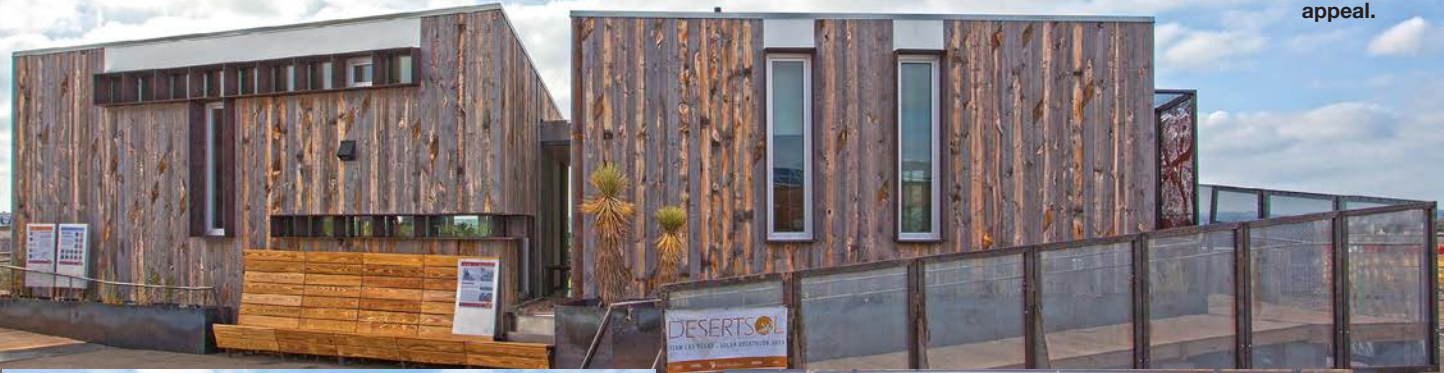
The south-facing PV awning also helps shade the doors and windows from the summer sun.
