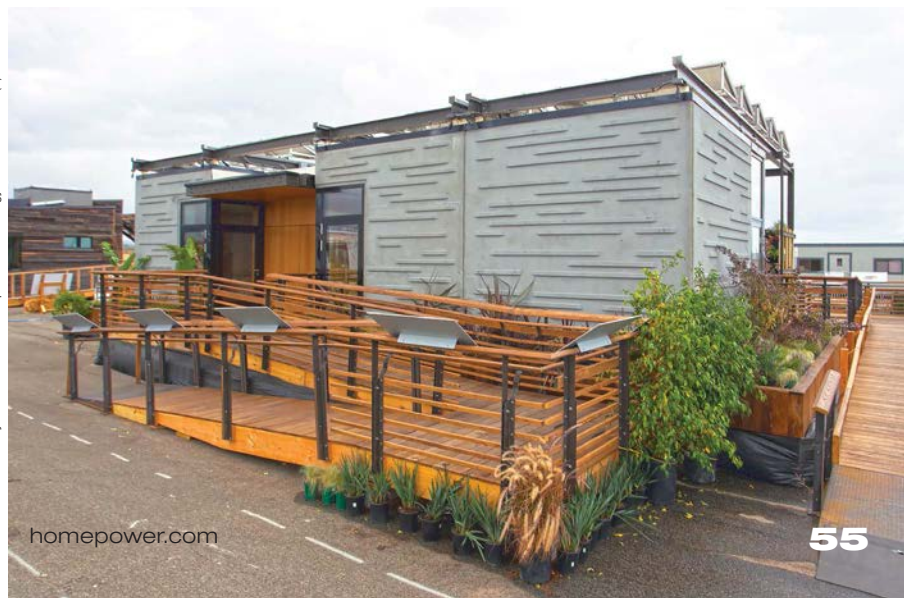
The precast concrete walls of UrbanEden, designed by students at the University of North Carolina, Charlotte, contain capillary tubes plumbed to roof-mounted flat-plate heat exchangers to allow heat transfer for heating and cooling.
