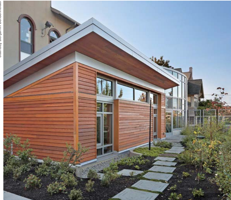
The LBC-certified Bertschi Living Building Science Wing in Seattle, Washington, met its Site petal, in part, by building on a former grayfield—a paved sport court.
