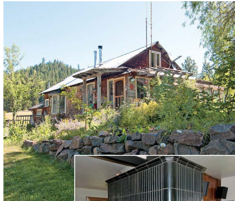
The 1920s farmhouse has been subject to several electricity upgrades.
