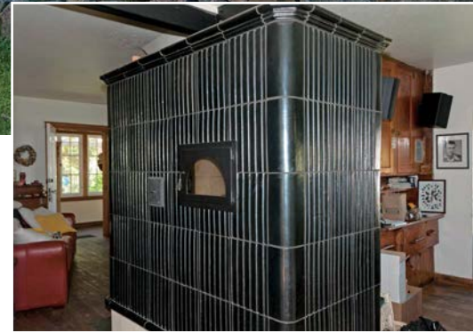
A central masonry fireplace provides efficient wood-fired heat all winter.
